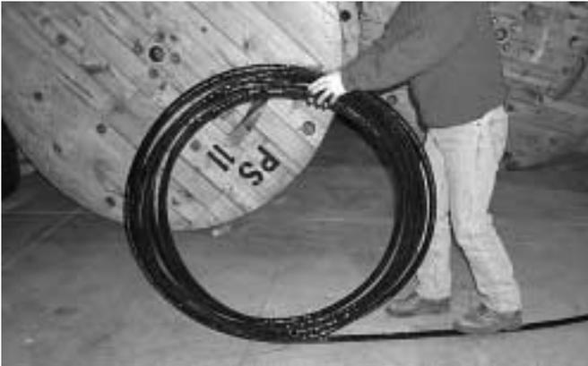
Method 2 - Use a second smaller spool to straighten the product as it is taken off of the larger shipping spool.
